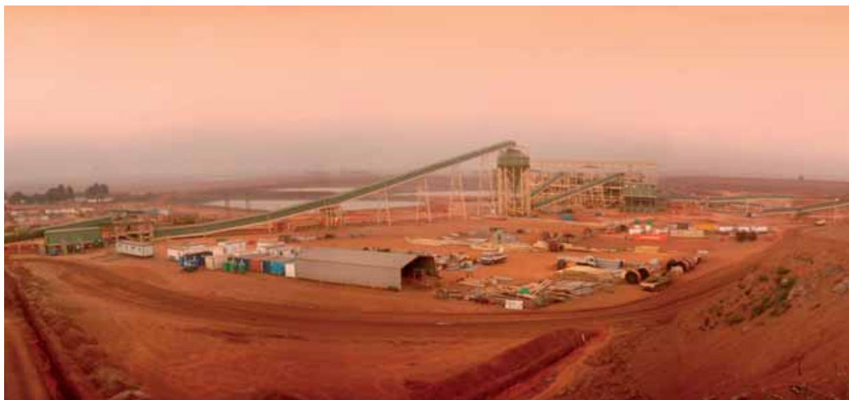
Coal washing and processing plant at Goedgevonden Coal Mine under construction
